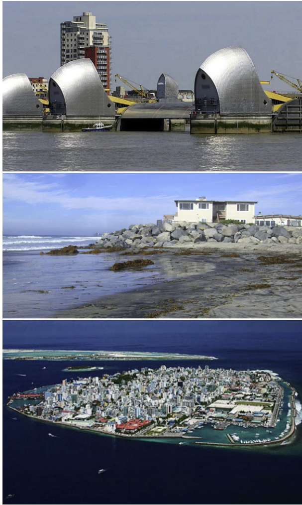
Figure 9 Examples of coastal protection and developments. Upper picture: the Thames Barrier, London, U.K., which is protecting more than 800 000 houses in the flood plane, including crucial infrastructure such as about 50 hospitals; Middle: Imperial Beach, California, where houses at a transgressive beach in a tsunami-prone area are protected with boulders, while the beach is transgressing past the developed coastline. Bottom: The island of Malé, capital of the Maldives Islands in the Indian Ocean. The maximum elevation is 2.4 m, and population is around 100 000. This extreme example of the hold-the-line (or even progression) strategy ( Figure 10 ) required a seawall around the entire island.
