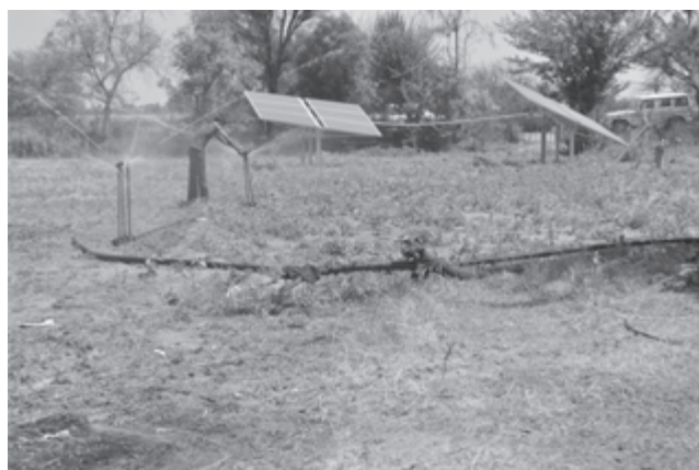
Photo 1. Micro-irrigation being energised by photo voltaic solar energy in India
